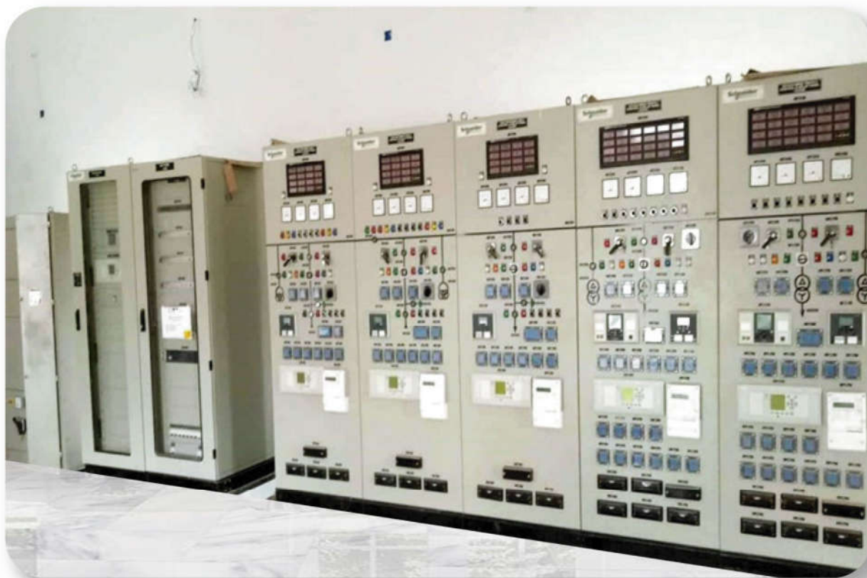
Newly Constructed 33/11 KV Control Room, Ghope, Jashore
