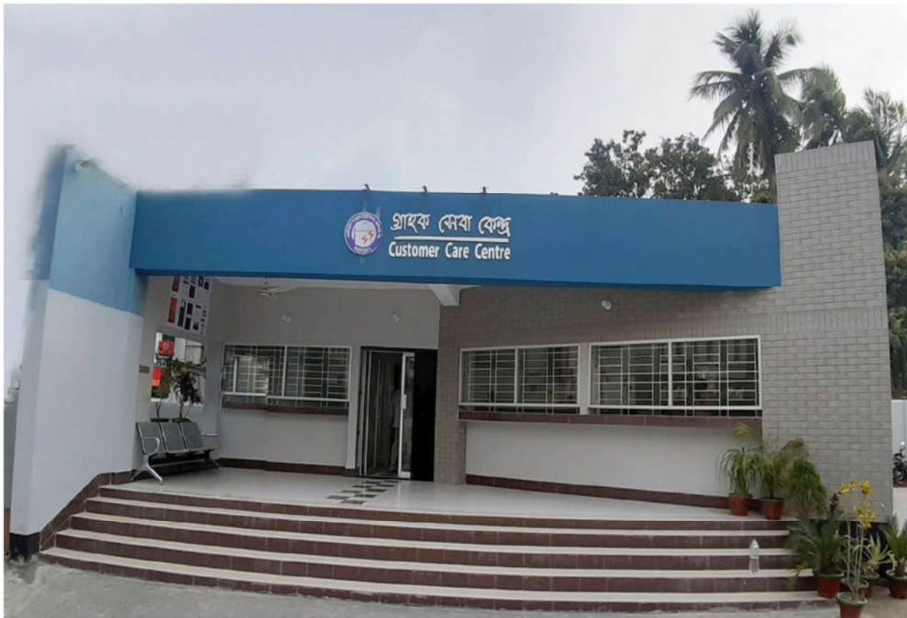
Newly Constructed Customer Care Center (CCC) At Jessore.
