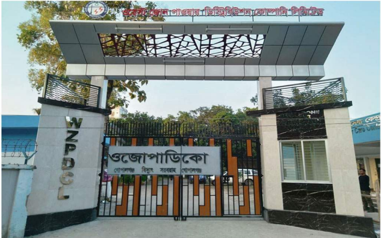
Newly constructed Main Gate of Gopalgonj ESU by EAPDSP
