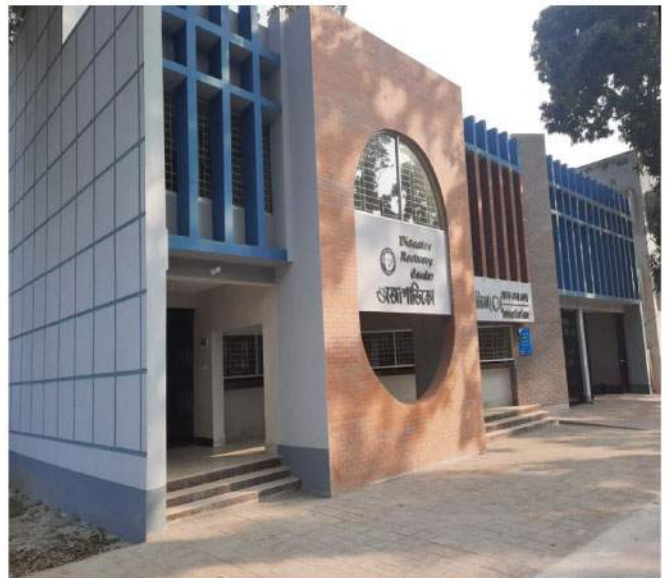
Newly Constructed Disaster Recovery Centre at Jashore
