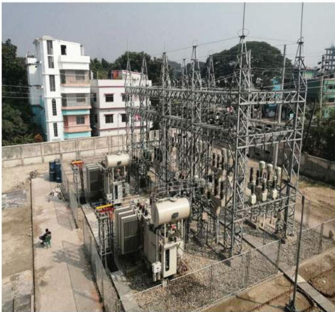
Newly constructed Jhinaidah Campus 33/11 kV, 2x10/13.33 MVA SS, Jhinaidah
