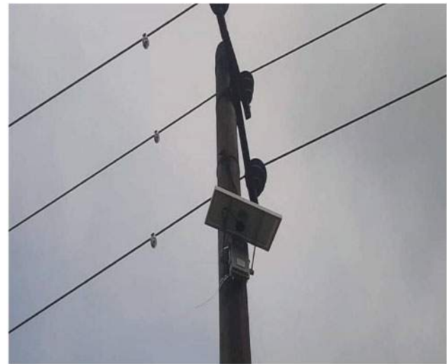
FPIs Installed in Patuakhali-Payra 33 kV Line
