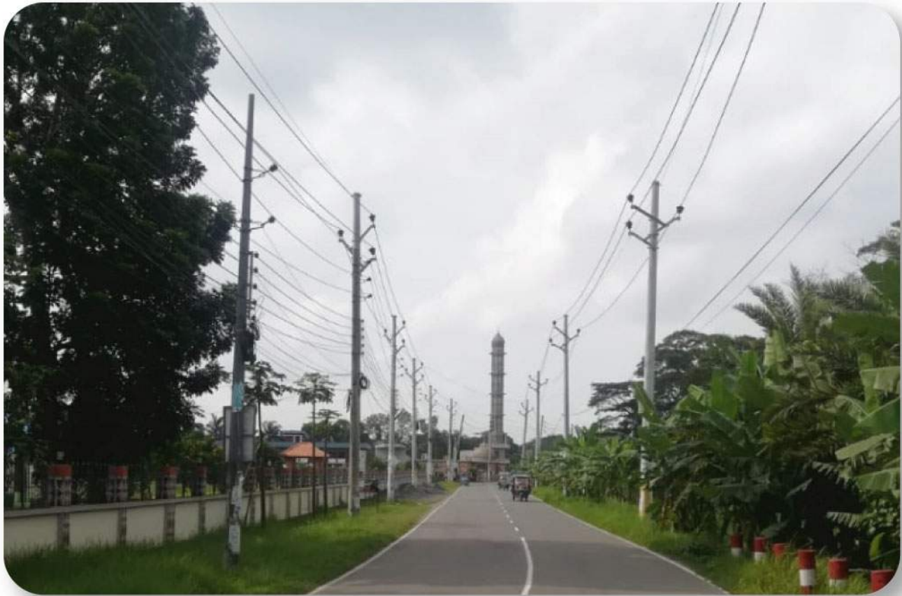
Newly Constructed Madaripur to Sariatpur Distribution Line Under WZPDCL
