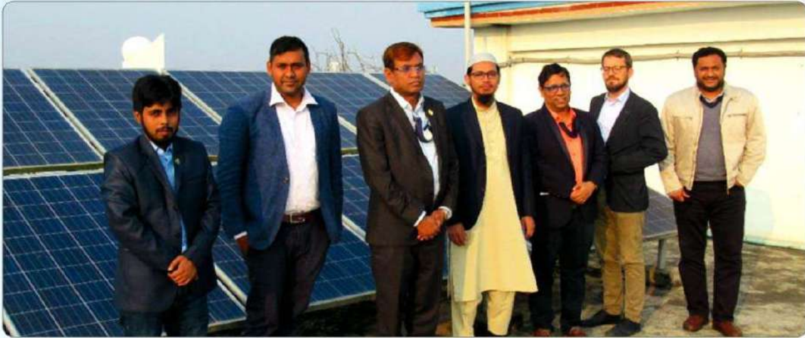
Net Metered Solar Rooftop at Gollamari in Khulna Fish Research Institute under WZPDCL Substation.
