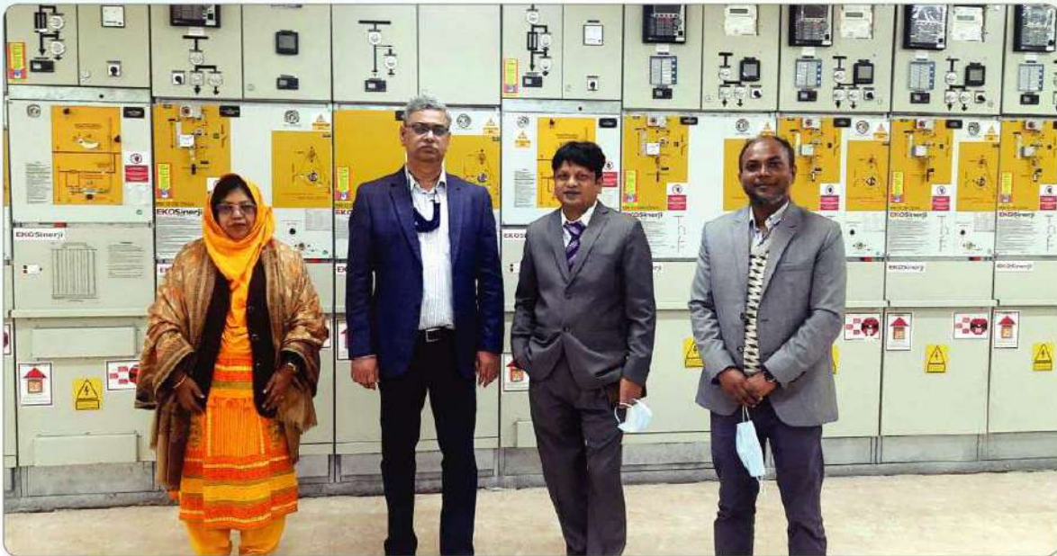
Sk. Munir Ahmed, Director (Management), Power Cell visiting newly constructed sub-station at Khulna
