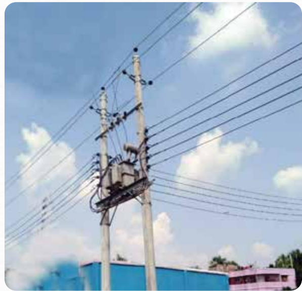
Newly Constructed Distribution Lines & Newly Installed Distribution Transformer under "Extension & Augmentation of Power Distribution System Project"
