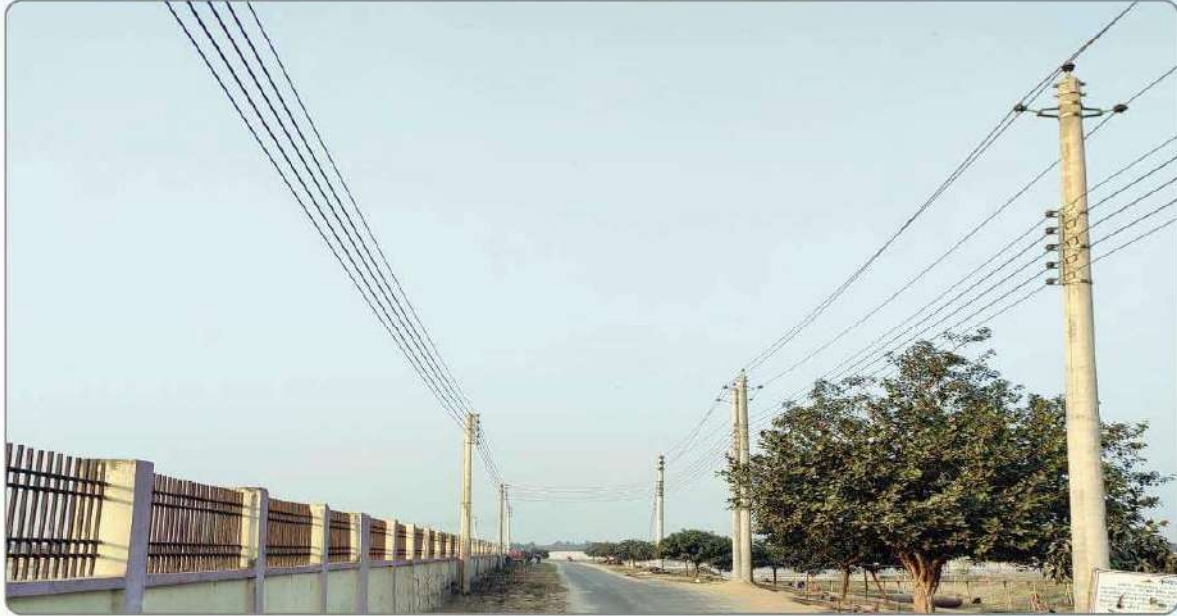
Newly Constructed 11/0.4 KV Distribution Line at Kushtia
