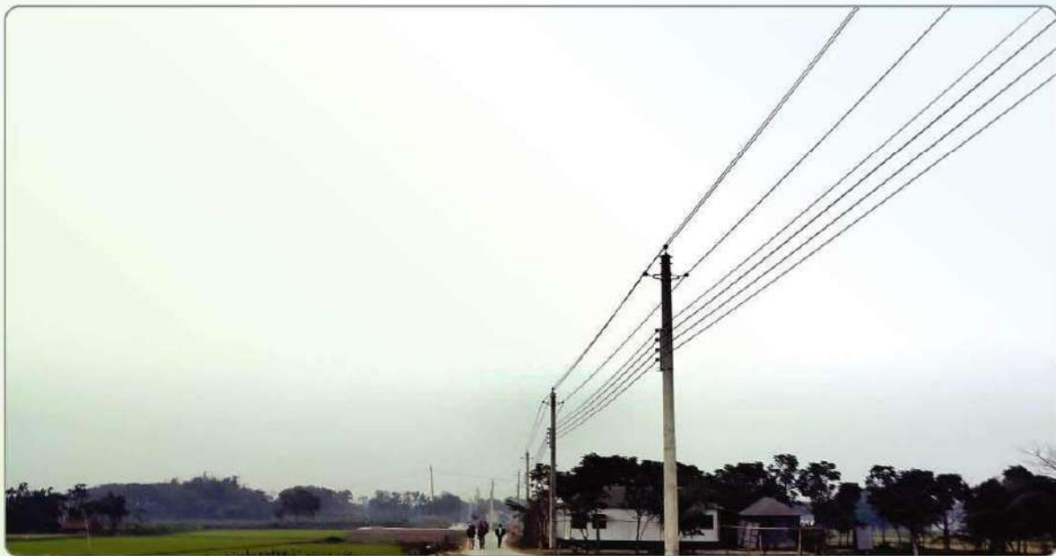
Newly Constructed 11/0.4 KV Distribution Line at Kumarkhali
