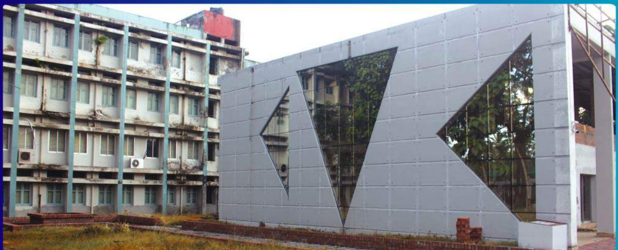
Lab Building, WZPDC Training Institute, Khulna.
